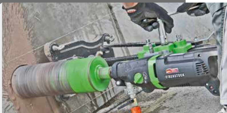
BST 182 V/S: mounted carriage on 4 special balls
